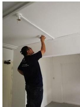
The HFAD will be installed on the ceiling of the living room within the HDB public rental flats. It will have to be installed somewhere in the middle of the living room, at least 3 metres away from the kitchen and away from any sources of smoke, so as to avoid false alarms. The HFAD installer will advise on a suitable location upon visiting the flat.
