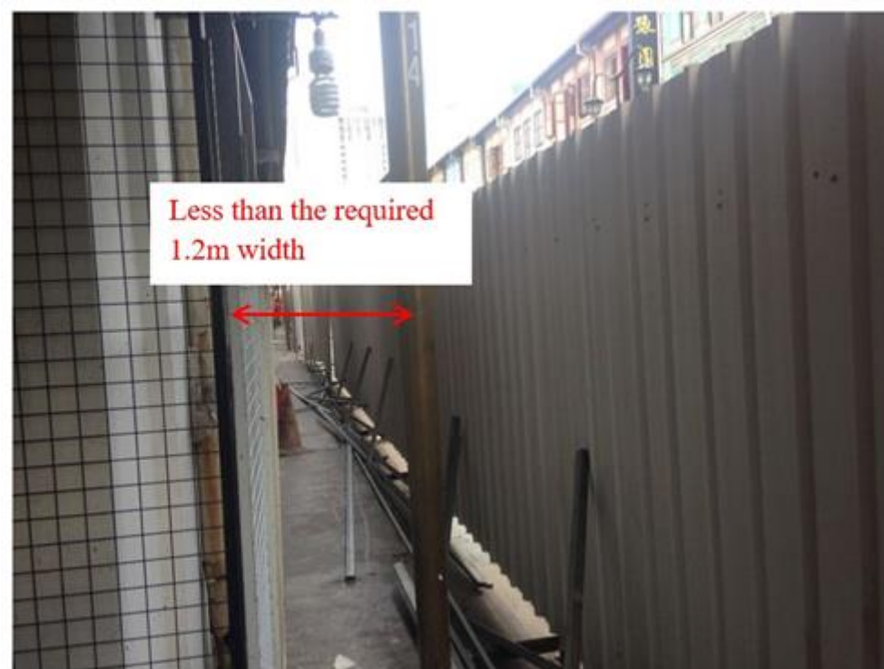
Diagram 9.9.4b.(2) - 1 : Hoarding obstructing means of escape
