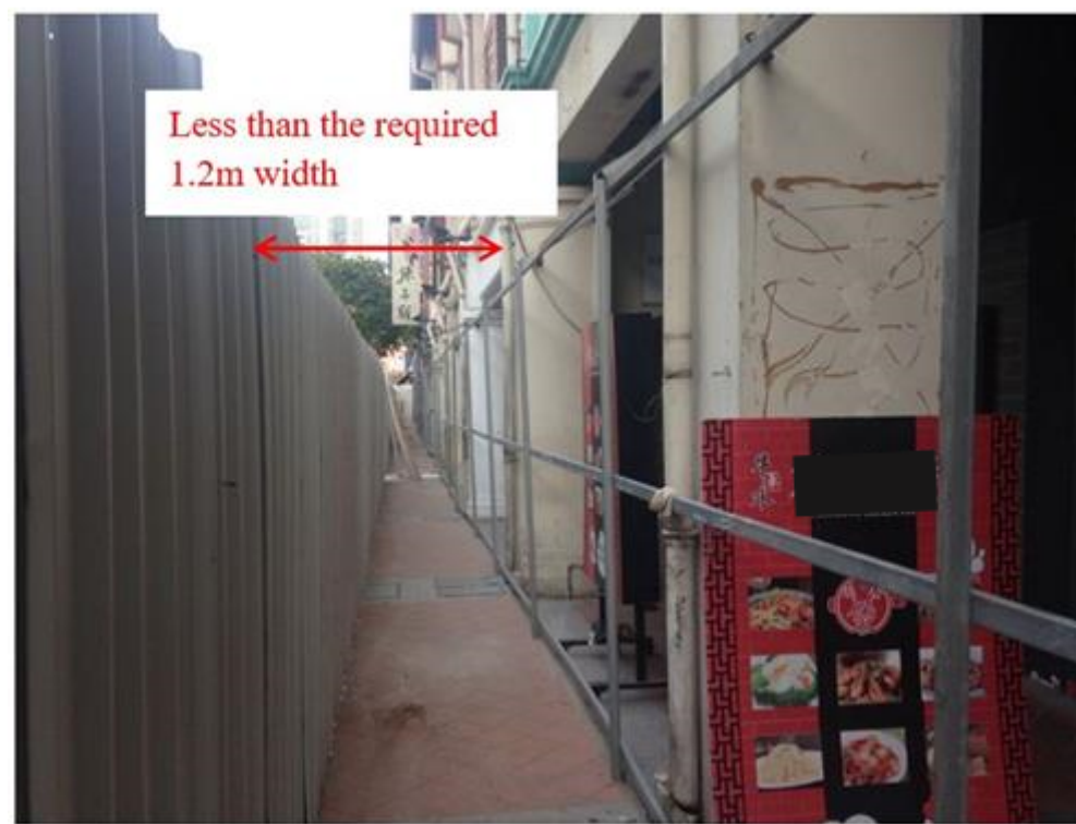
Diagram 9.9.4b.(2) - 2 : Hoarding obstructing means of escape
