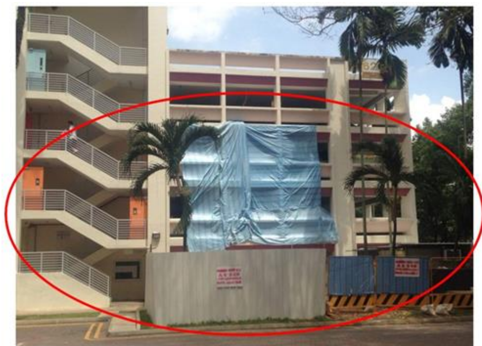
Diagram 9.9.4b.(2) - 4 : Hoarding obstructing openings for smoke dispersal
