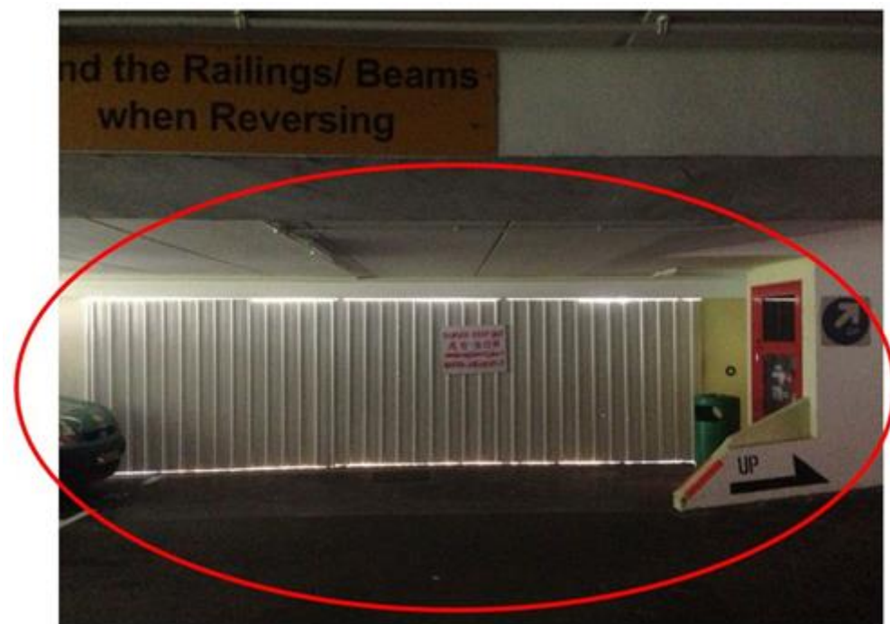
Diagram 9.9.4b.(2) - 3 : Hoarding obstructing openings for smoke dispersal
