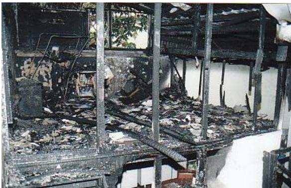
**Figure 12. Fire developed and burned into the rooms**
