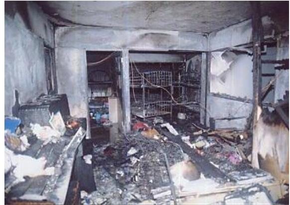
**Figure 11. The fire consumed the wooden partition and spread into the living room**
