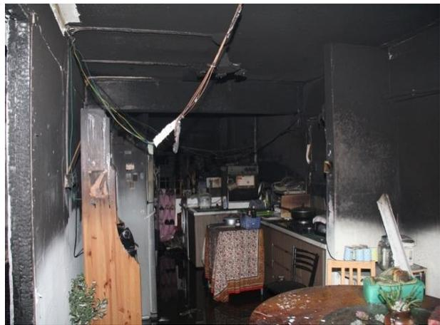
**Figure 21. Other parts of the residential unit sustained heat and smoke damage**
