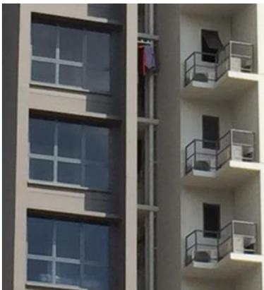
**Figure 2. Condensing Units on A/C ledges**
