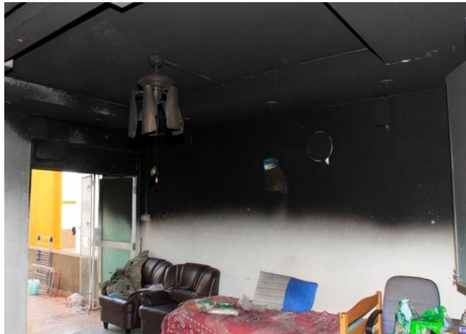
**Figure 19. The apartment sustained heat and smoke damage as a result of the ceiling plume from the FCU fire**
