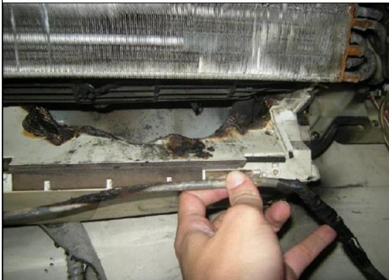
**Figure 25. The burnt area on the FCU with the electrical cable that was running across**
