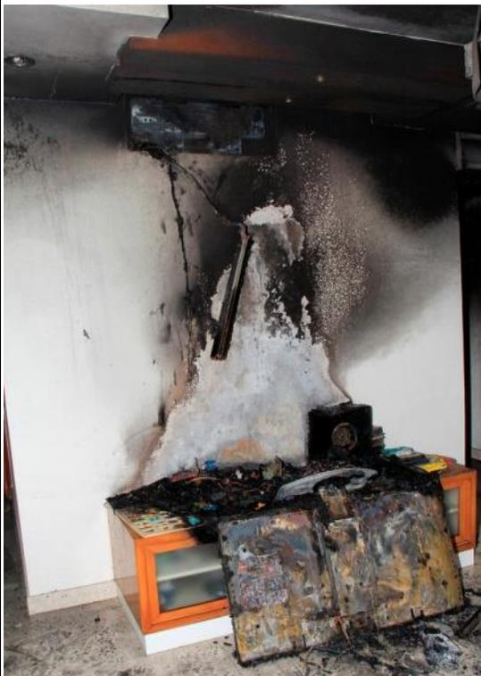
**Figure 18. Drop down from the FCU fire damaged the TV and other items beneath**
