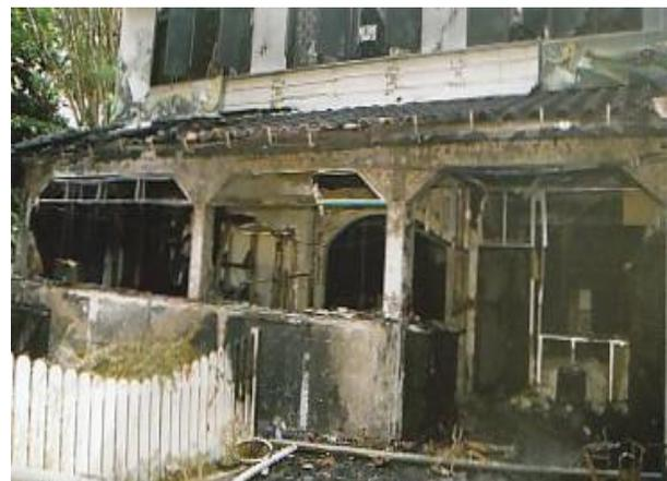
**Figure 17.** Other parts of the building sustained heat, smoke and water damage
