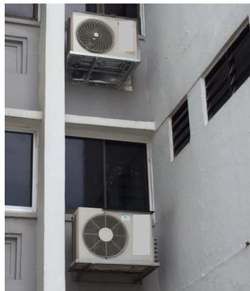
**Figure 3. Condensing Units on brackets**
