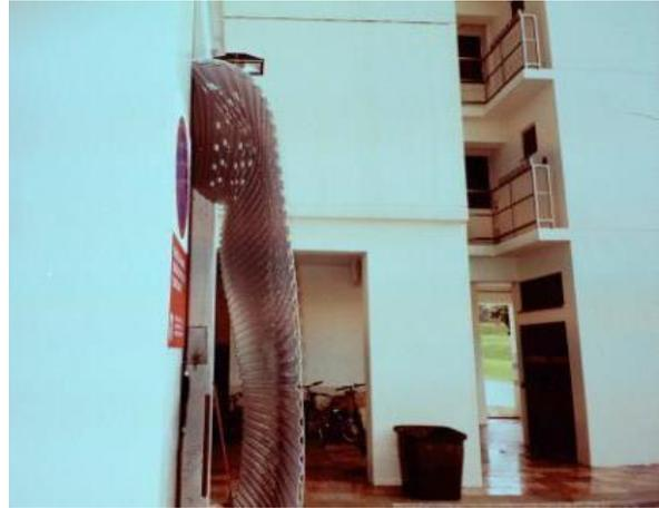
**Figure 14. The damaged roller shutter**
